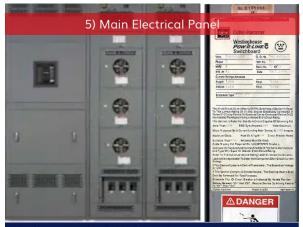
Showing us the data plate for the main gear can help us identify cabinet manufacturer, make, model, and type so we can correctly select breaker size and type if one is needed.
