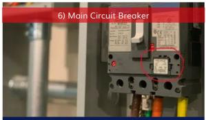
Main breakers come in many shapes and sizes. Please ensure that we can see the rating of the breaker and the set points in the form of a rating plug.
